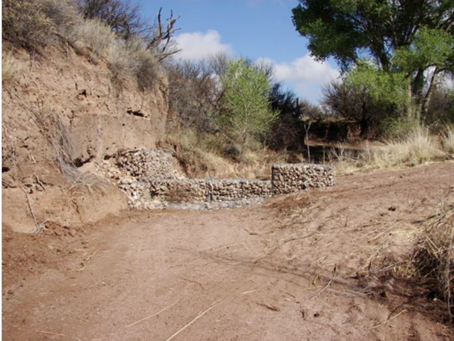
Gabion 3 – March 2009. Photo taken looking north. The west side of the gabion is flush against the tall bank.
