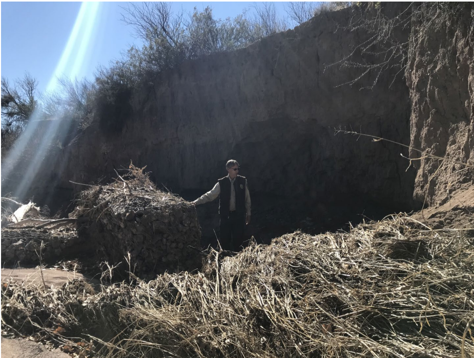
Gabion 3 – January 2020. Photo taken looking south. Due to the significant pulse of water released upstream, the bank on the west side of the gabion eroded significantly.
