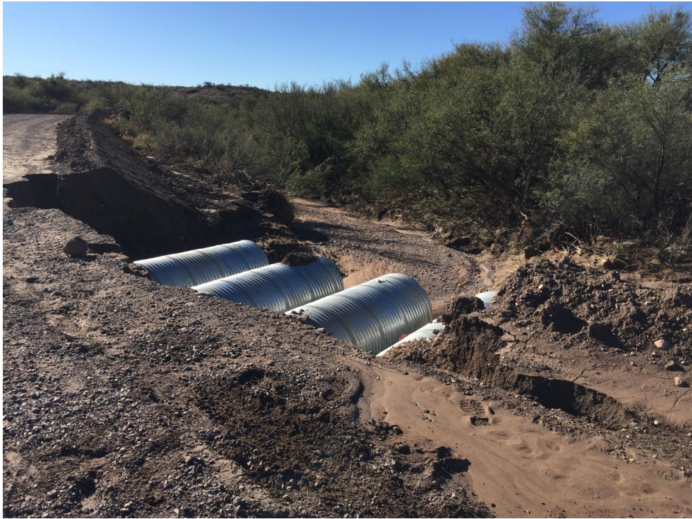
Picture 1. November 2019. Post flood event blow out of Hay Hollow Crossing
